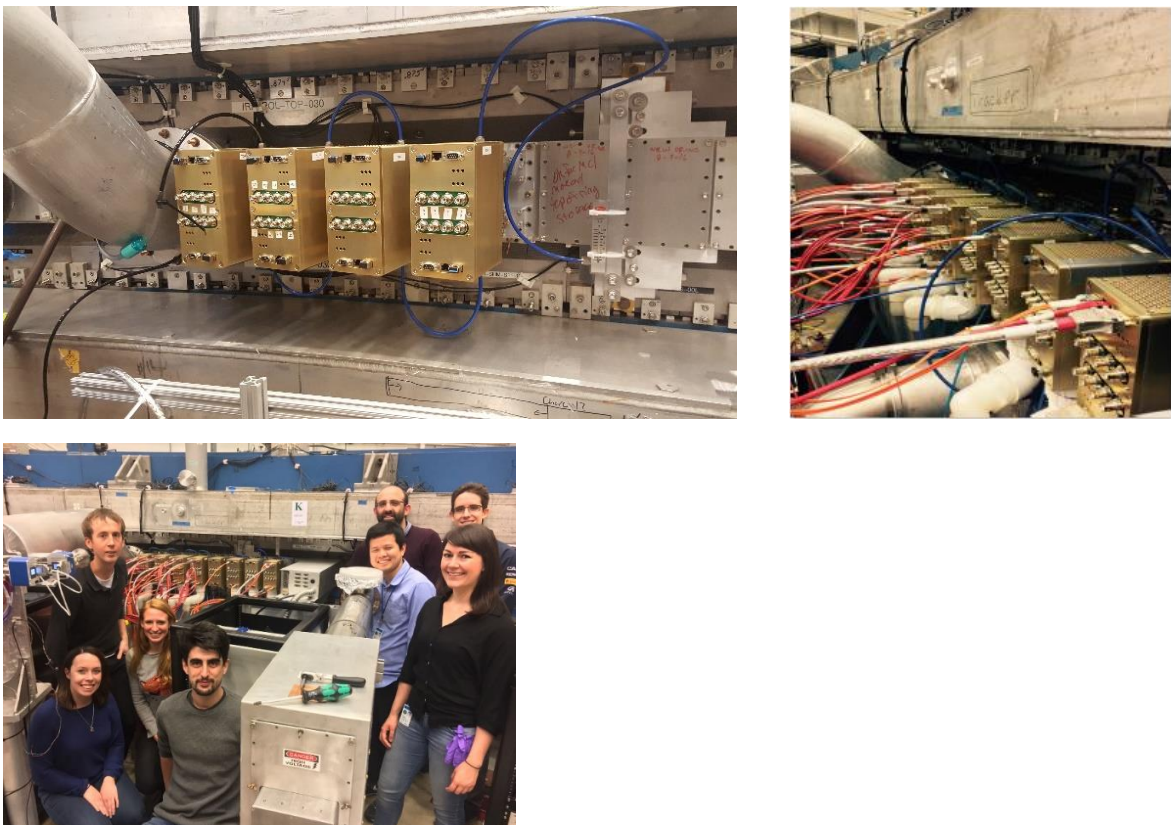
Figure 27: Installation of the first complete tracker prior to the 2017 Commissioning Run.
