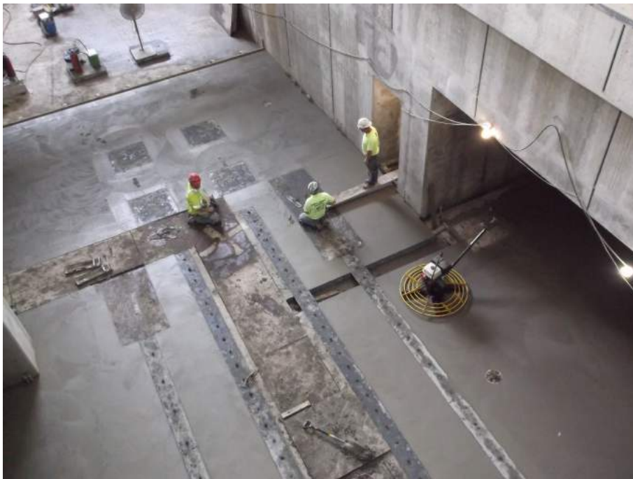
Figure 7.14. Looking down on the Mu2e detector hall. Equipment alcove A is to the right. Towards the top of the picture within the alcove, a square outline of the DT generator bunker is visible, with a trench extending out to the hall and another trench following the top wall of the alcove. There is a larger covered longitudinal trench connected where the source trench terminates near the center of the hall.
